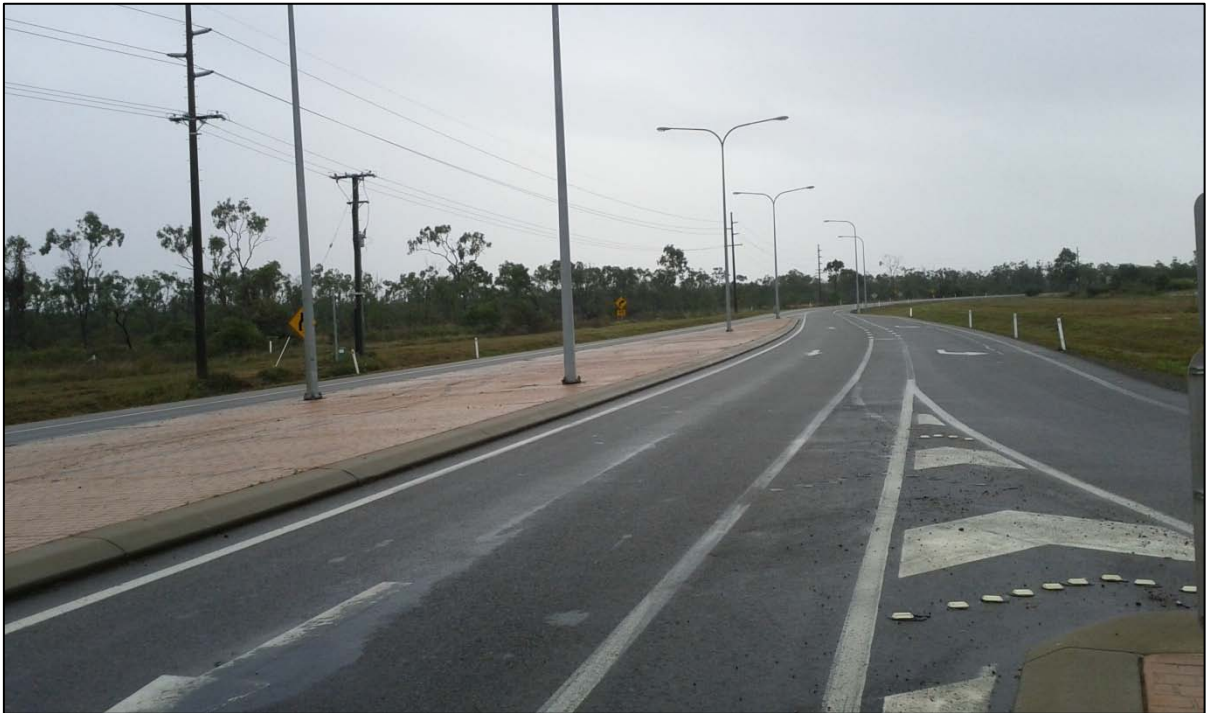
Figure 2.4 Shaw Road looking north past the subject site
