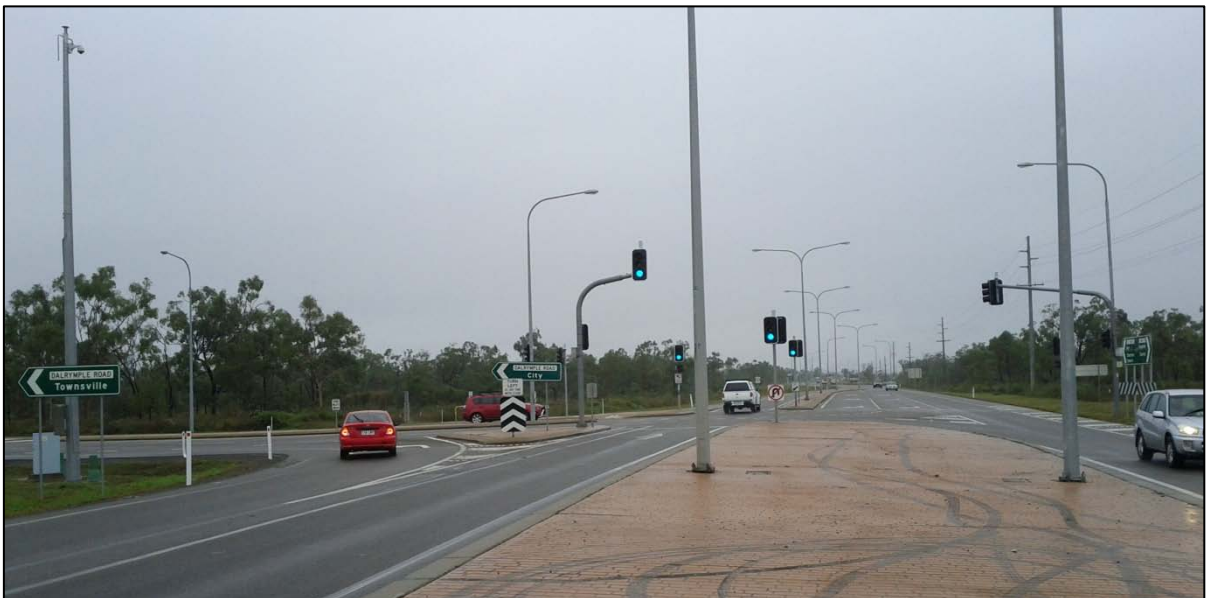
Figure 2.6 Shaw Road / Dalrymple Road / the Ring Road intersection looking south from Shaw Road
