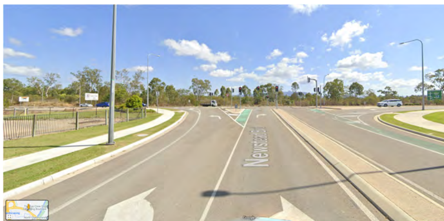
Figure 8 – Hervey Range Road and Hogarth Drive Intersection (Google Maps)
