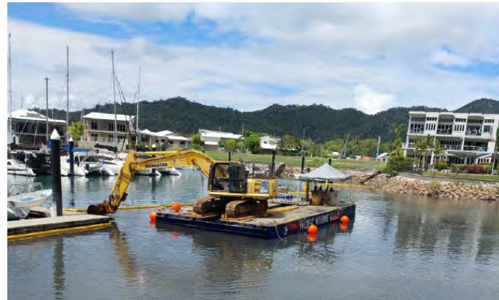
14m x 7m pontoon with 20t excavator onboard which will be used where space is limited
