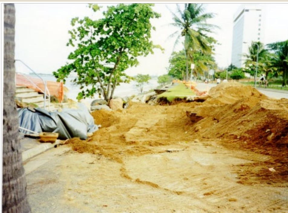
Unknown (1998), Damage to the Strand, Townsville, 15th January 1998.
