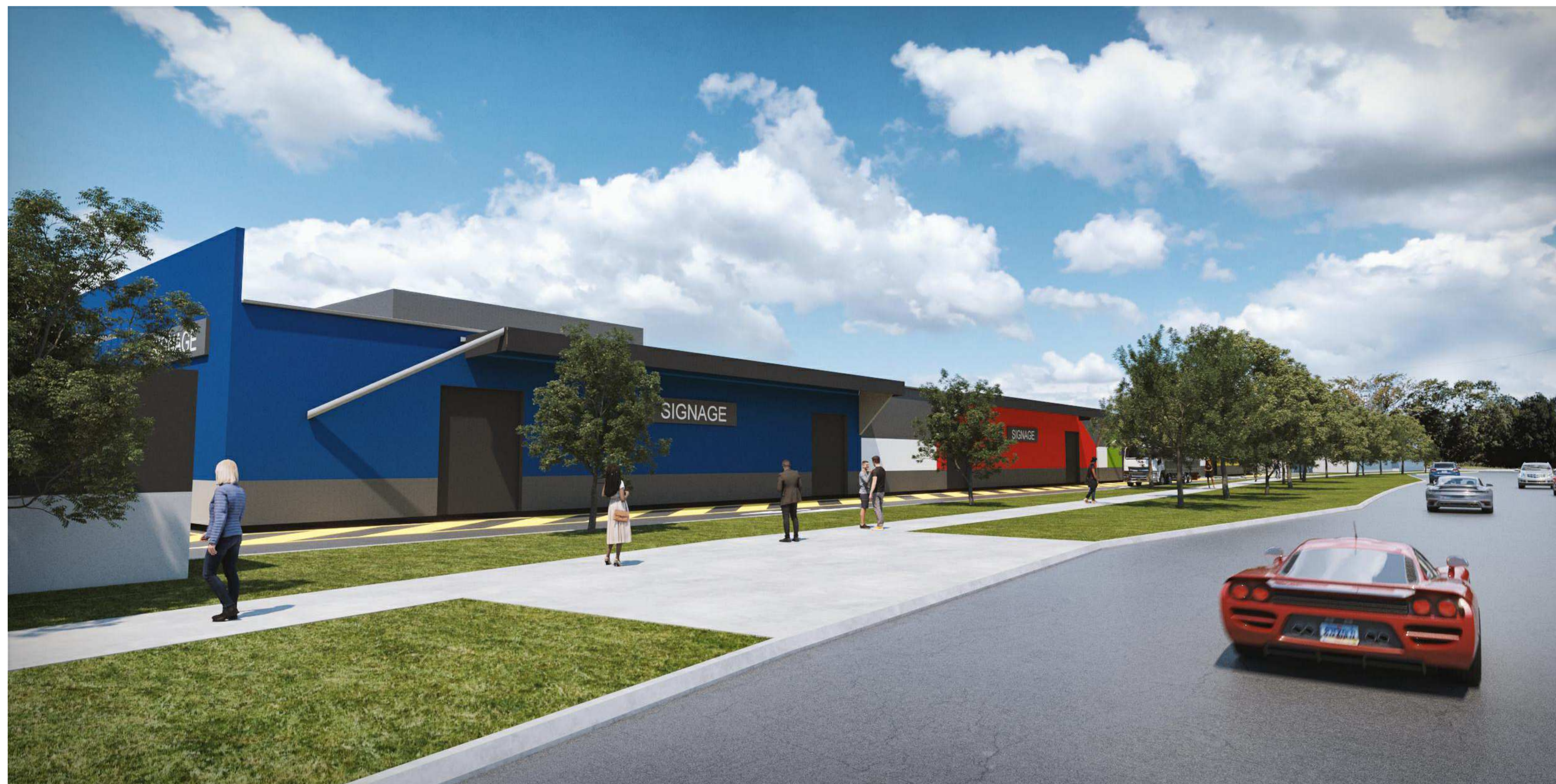
VIEW 5 - VIEW FROM NORTH SHORE BOULEVARDE
