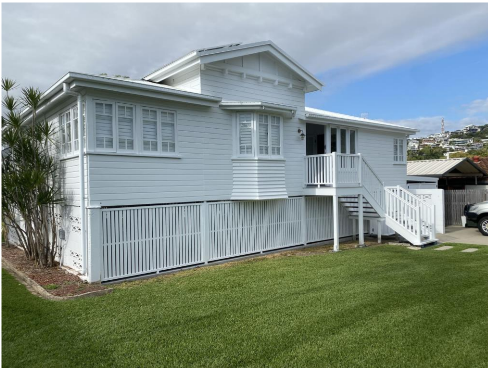
Figure 1 - Existing Residential Dwelling
