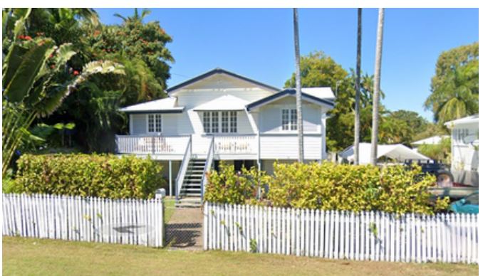
Adjoining Lot - North
