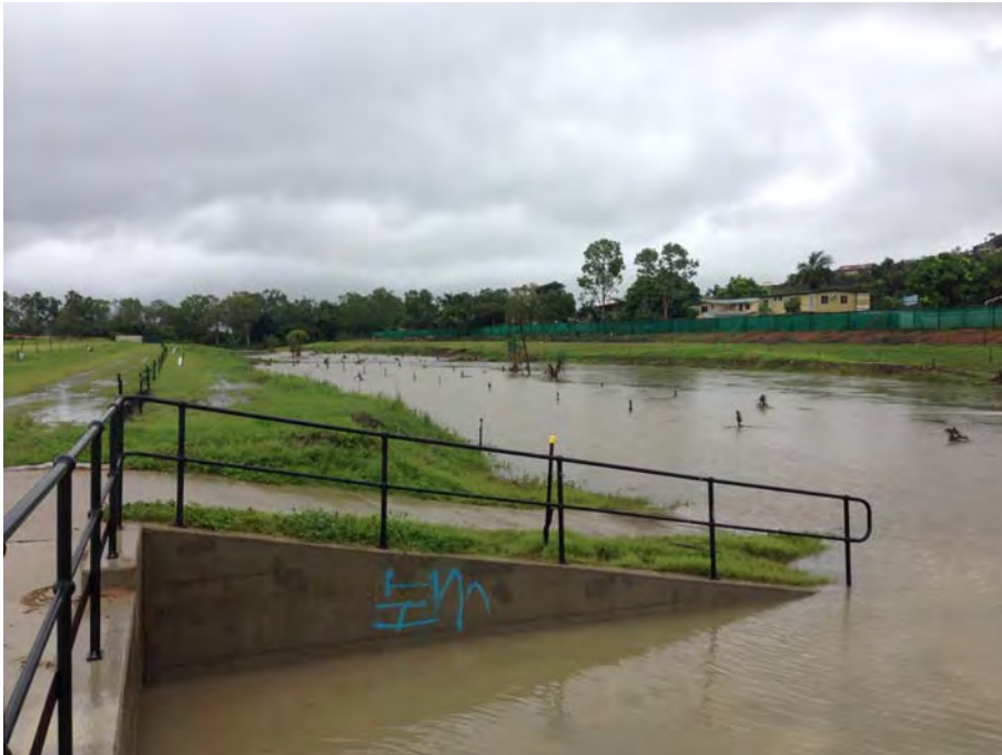
Photo 10 – Louisa Creek Diversion Channel at 10.30 AM on 13 th Apr 2014
