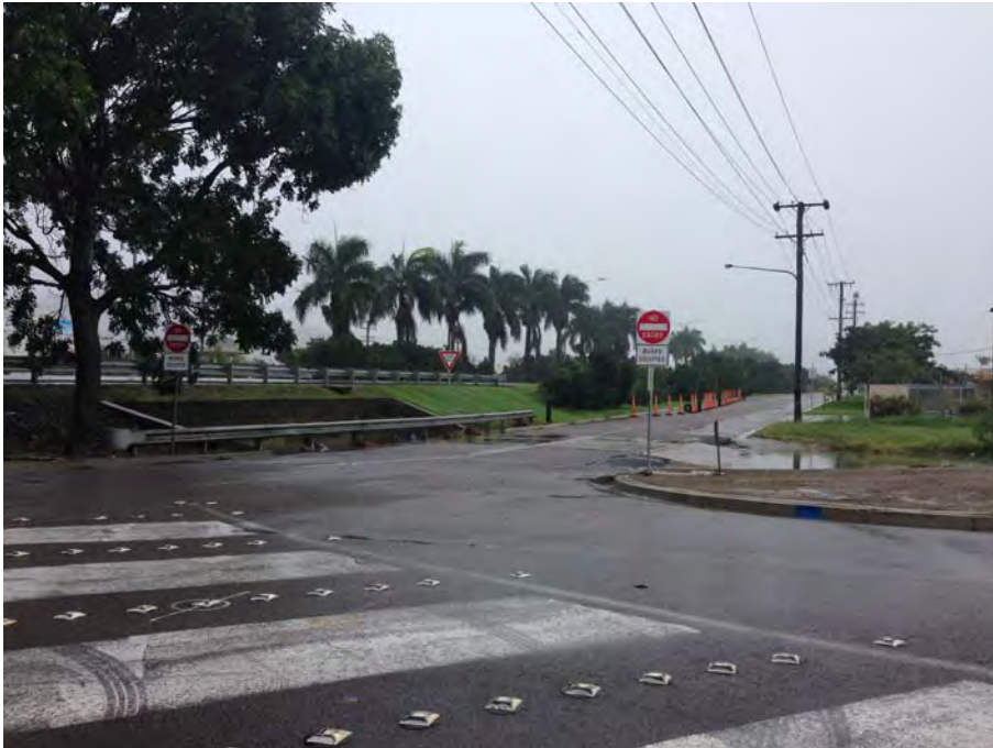
Photo 12 – Pee Wee Creek downstream of Woolcock Street at 09.37 AM on 13 th Apr 2014
